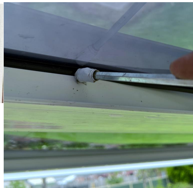
Use a round edged piece of wood or plastic to hit or push the rubber into the groove.
