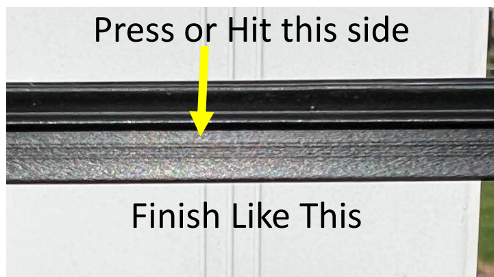
Use a round edged piece of wood or plastic to hit and push the rubber into the groove.
