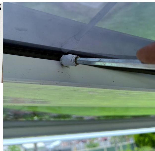
Use a round edged piece of wood or plastic to hit and push the rubber into the groove.
